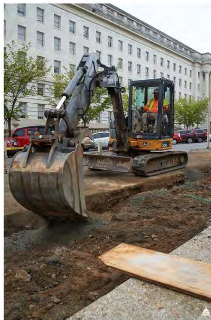
The House's Cannon HOB subsurface infrastructure being rebuilt, 2019. Photos: AoC.
